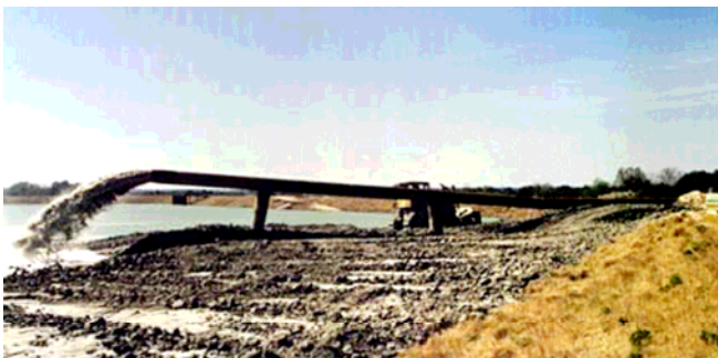
Florida Inland Navigation District Dredge
